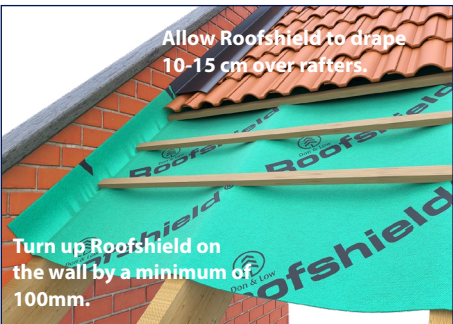
Side Abutment Detail
