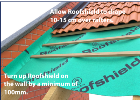
Side Abutment Detail
