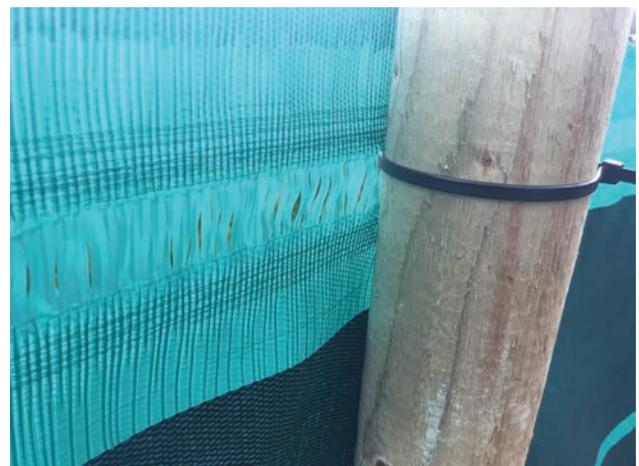
*Specially designed vented area for easy fixing to fence posts*
